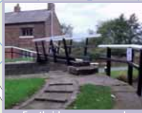
Footbridge across canal
